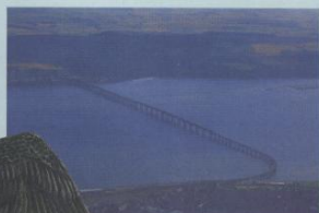
The Tay Rail Bridge forms the eastern boundary of the Inner Tay Estuary.
