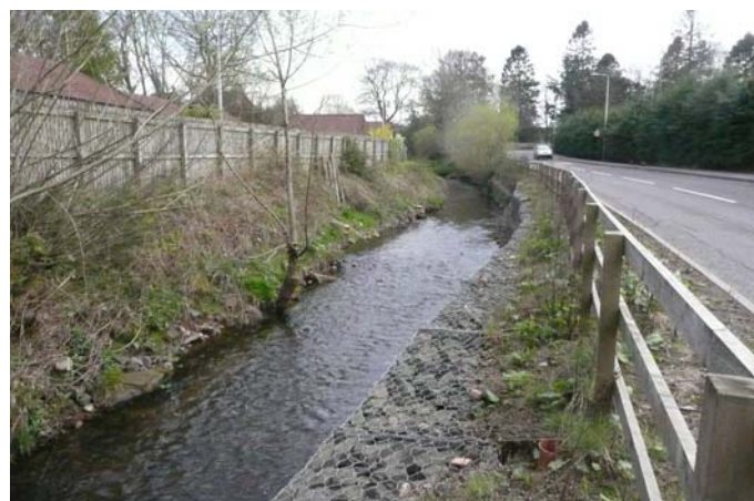
View 16: East Pow Burn erosion protection at Lochty Park.
