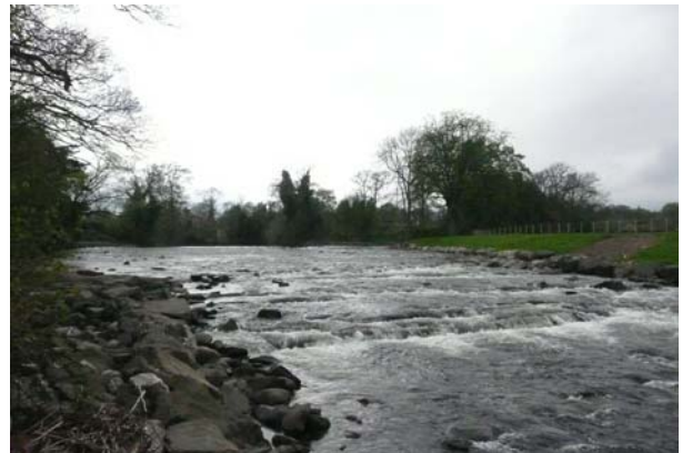
View 10: River Almond erosion protection, left bank at Low Works Weir.
