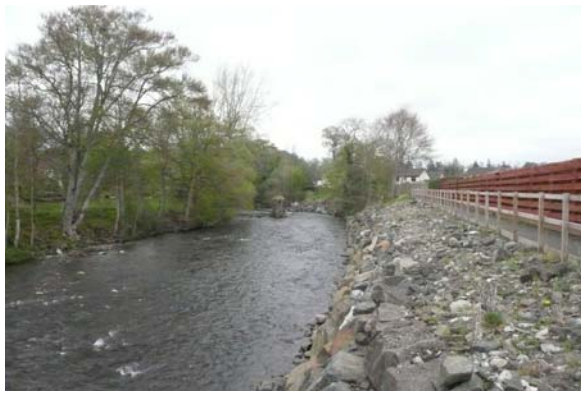
View 9: River Almond erosion protection, right bank adjacent to Almond Grove.
