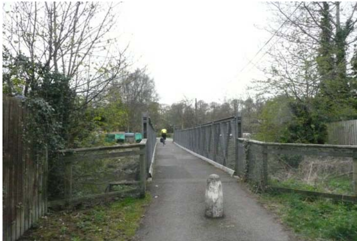
View 14: Existing Footbridge.
