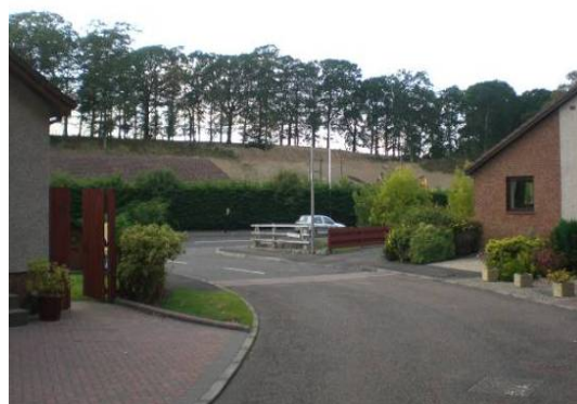
View 18: Lochty Industrial Estate September 2009 - major works to sloping bank.
