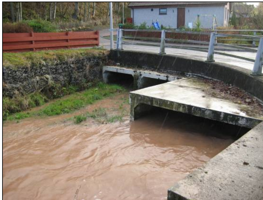
Figure 17 – Lochty Park Road Bridge
