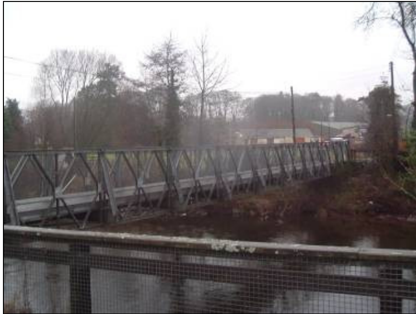
Figure 15 – River Almond Footbridge
