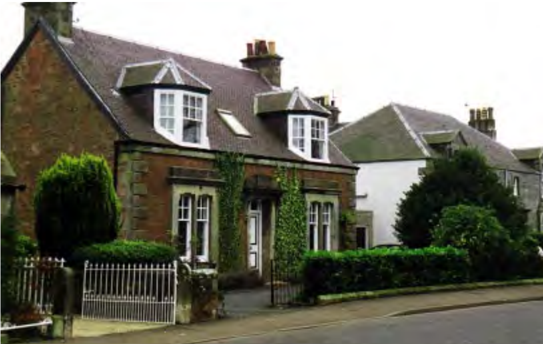
A detached stone house, with Dormers permitting accommodation in the roof space - Kinross. Note :Stone division walling, railing and hedging used together.
