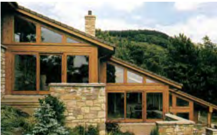
Successful combination of timber, glass and natural stone for housing at Kinfauns, Perthshire. Architects: McLaren, Murdoch and Hamilton.
