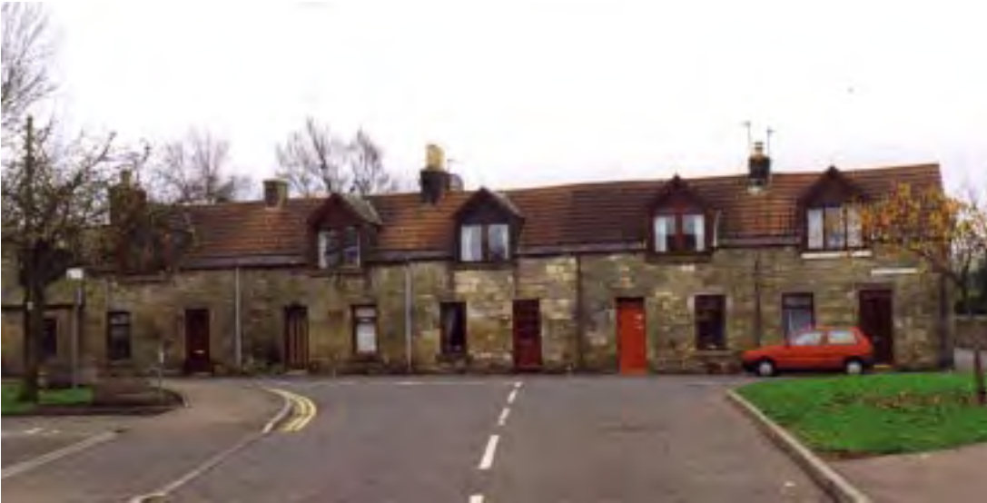
A Terrace of stone built Cottages at Kinross.
