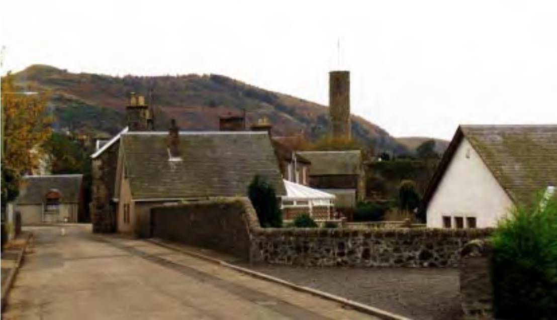
The round tower as a focal point at Abernethy. Note how the stone boundary walls tie the buildings to the ground.
