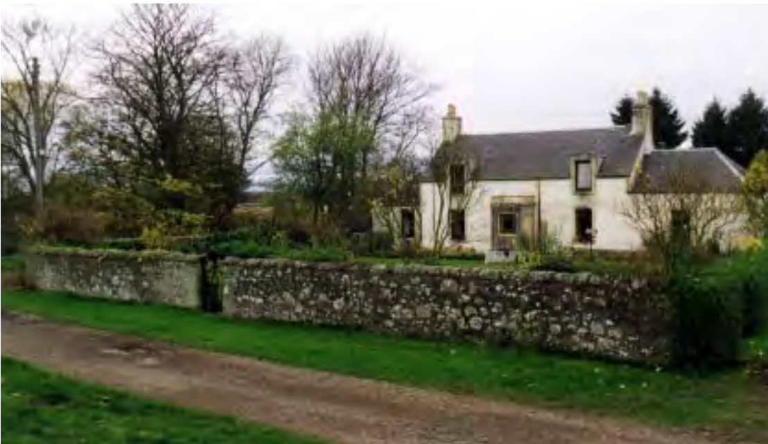
A detached house at Aberargie using slated roofing with white roughcast and stone banding around the windows. The private garden space is defined by stone wall, gate and hedging.
