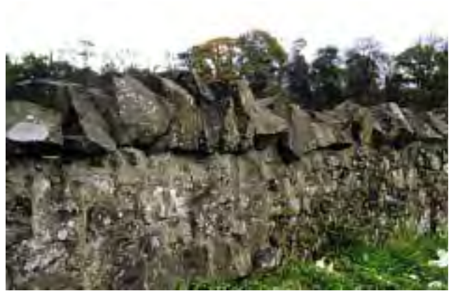
Stone wall along B935 Using field stones, rough coping
