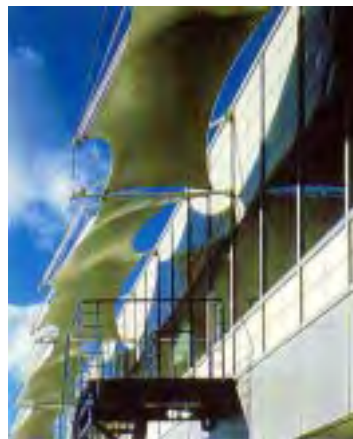
Office and Administrative unit at Stockley Park, London. Architect: Troughton Macaslan
