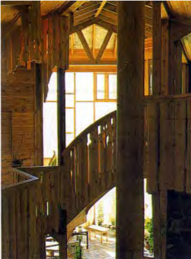
House at Stavanger, Norway. Built of timber and other organic materials, this house has transusive walls that allow it to breathe. Architect: GAIA Architects Group
