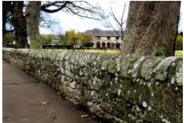
Low stone wall alongside bowling green, Kinross Semi-circular coping
