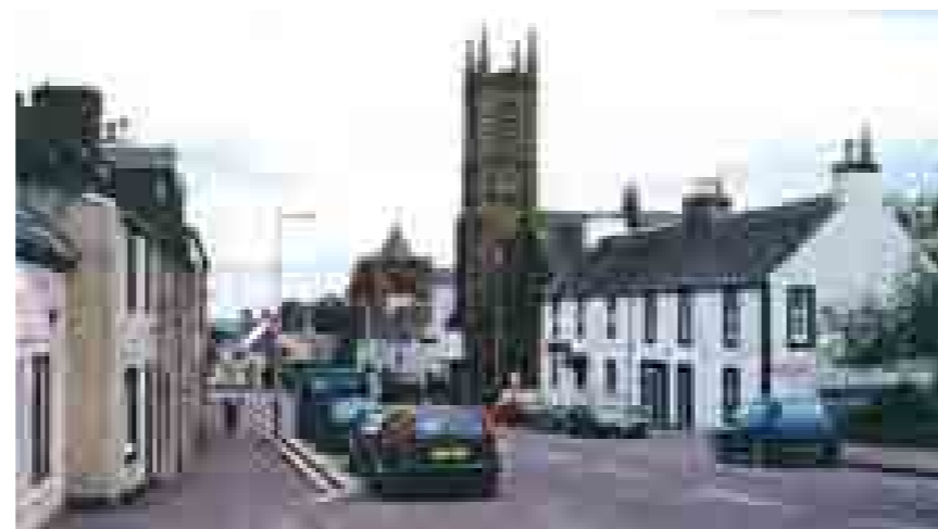
Figure 11. High St. looking east with Barony Church and Former free church on right
