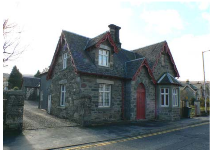
West Toll House (The Armoury), Kenmore St
