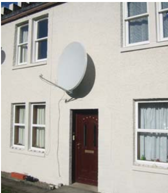
Oversized satellite dish on main façade
