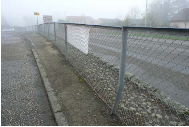
Metal barrier fencing, Back Dykes
