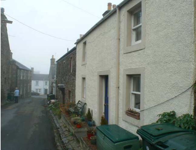
Terraced houses and setted open drain, Kirk Wynd
