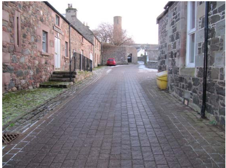
Unsympathetic concrete block paving
