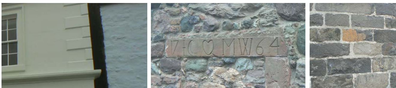
Painted ashlar and rubble in subtle tones, decorative marriage lintel and coursed whin stone
