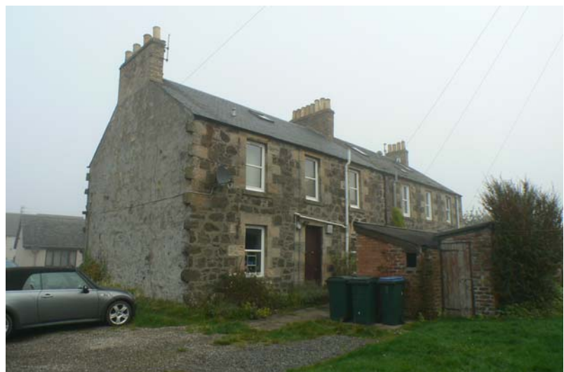
Back-to-back tenement building, Bank Buildings, Back Dykes
