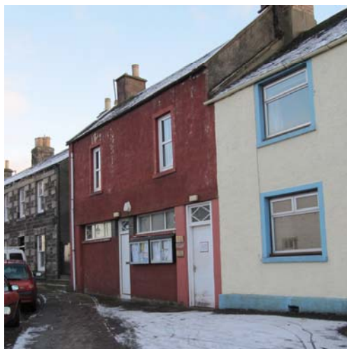
Altered façade, Main Street
