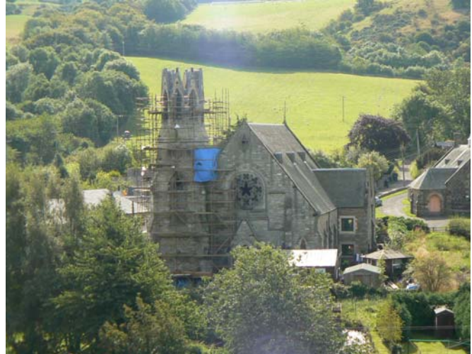
Former church with reduced steeple, photo taken from Round Tower in 2007
