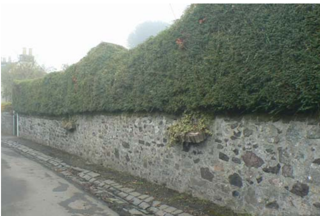
Traditionally built rubble wall with hedging
