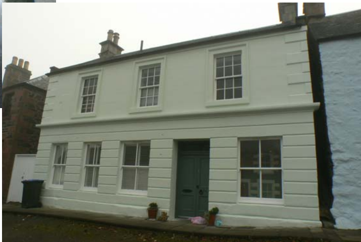
Early 19th century building with classical features such as ground floor channelling, angled quoins and window architraves at first floor
