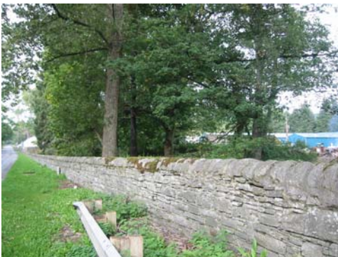
Distinctive use of rubble and dressed stone, slate and timber.
