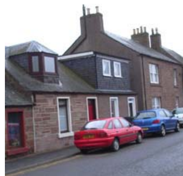
Poor dormer design
