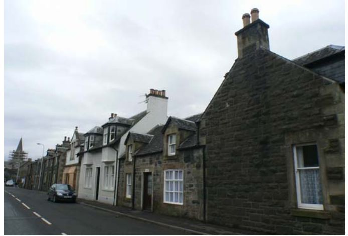
Variety of dense housing in Dundas Street
