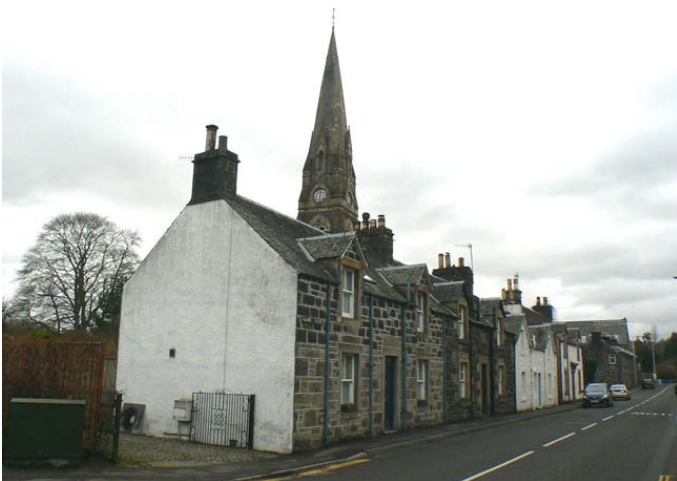
Burrell Street with impressive spire of Comrie and Strowan Parish Church in background
