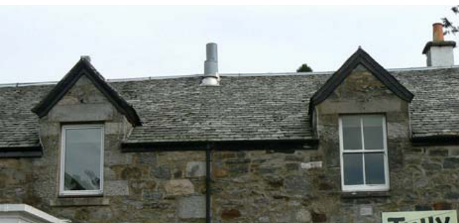
Original window to the right and non-traditional replacement window to the left within the same building
