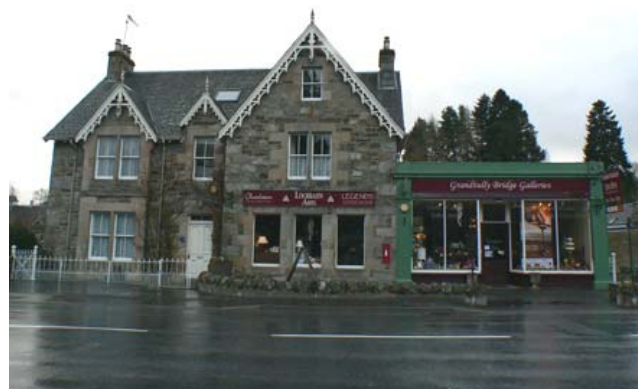
Grandtully Bridge House
