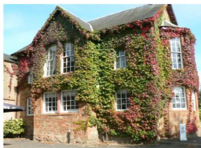
Inchtute Hotel: Historic landmark and listed building
