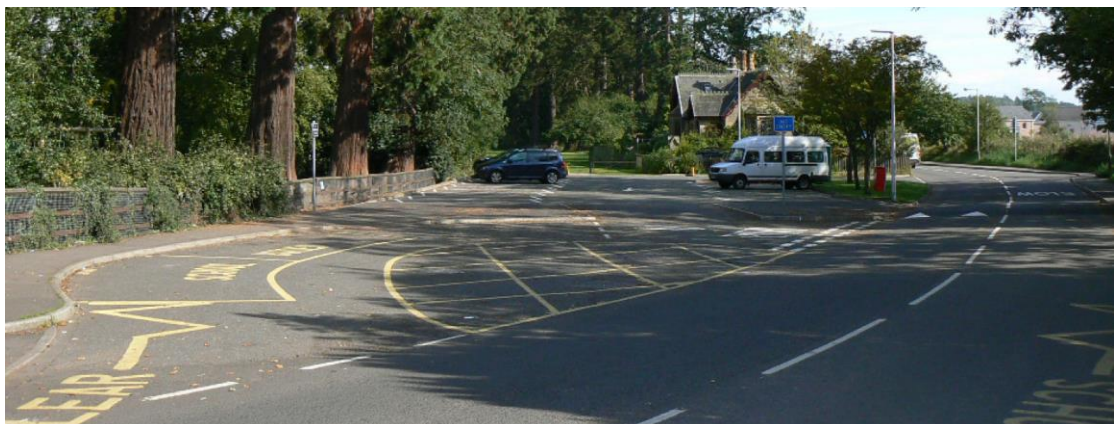
Tarmacadam area which would benefit from physical boundary treatments to enhance the conservation area and mitigate road user confusion.
