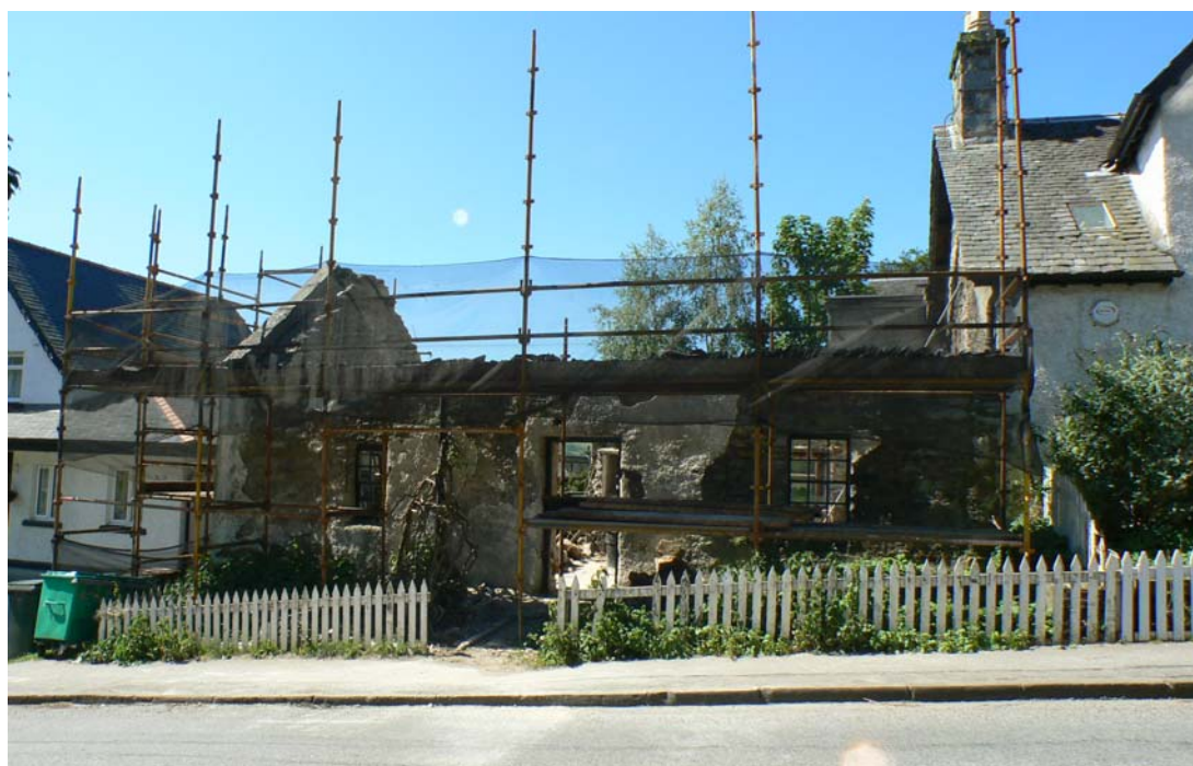
Deuchars Cottage, restoration in progress
