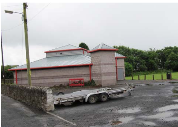
Myre Terrace, changing room building
