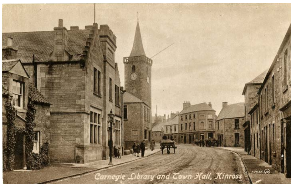
High Street, looking north, c.1935
