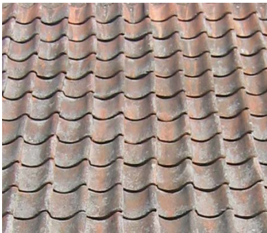
Traditional pantile roof
