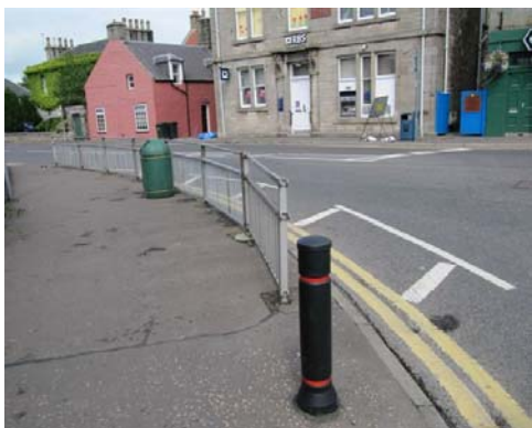
Standard bollards and barriers
