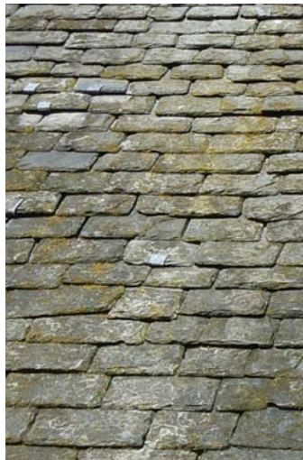
Traditional slate roof
