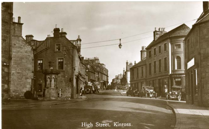
High Street, looking north, c.1930
