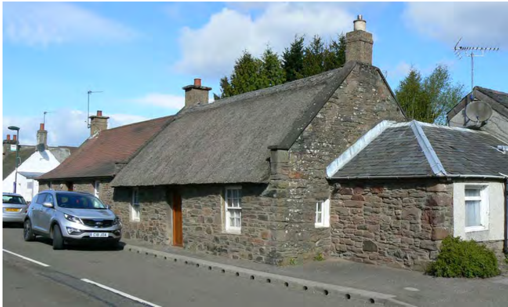
Steeple Cottage and The Quoins, Main Street
