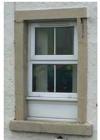
Example of an inappropriate replacement window
