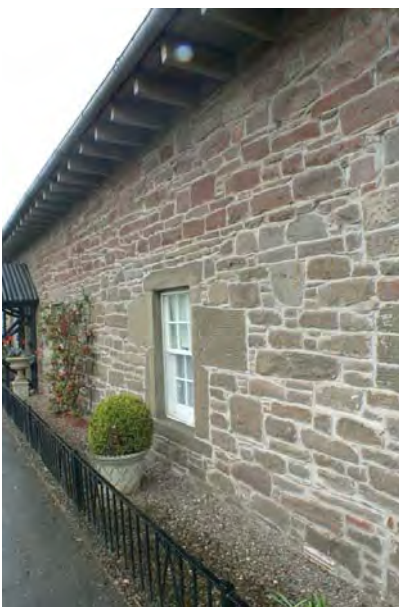
The Cottage, wallhead heightened
