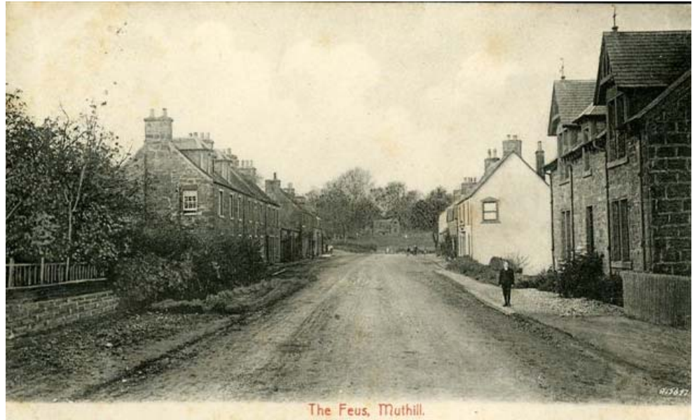
Entrance to Willoughby Street from the south east (Braco), date stamp 1915
