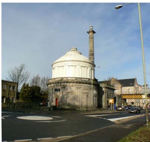
J.D. Fergusson's gallery, former waterworks
