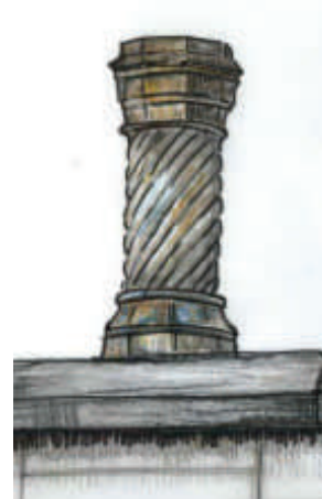
Ornamental chimney can
