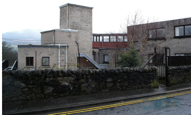
Rear elevation of Scotland's Hotel
