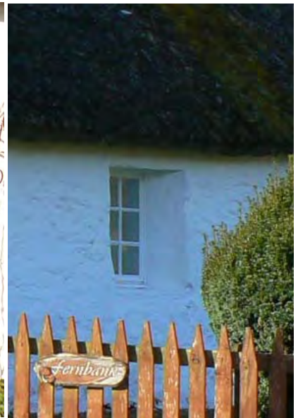
Small window opening, with frame set deep into the thick walls
