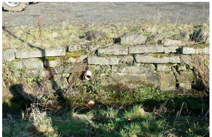
Low stone built retaining wall to sides of burn
