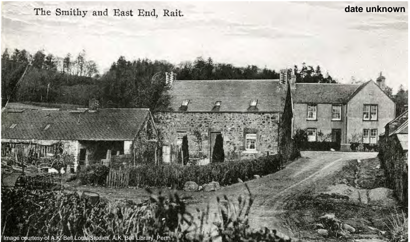
Historic photo showing the Smithy (far left), Smithy House (central) and former Inn/Little Rait farmhouse in the background
