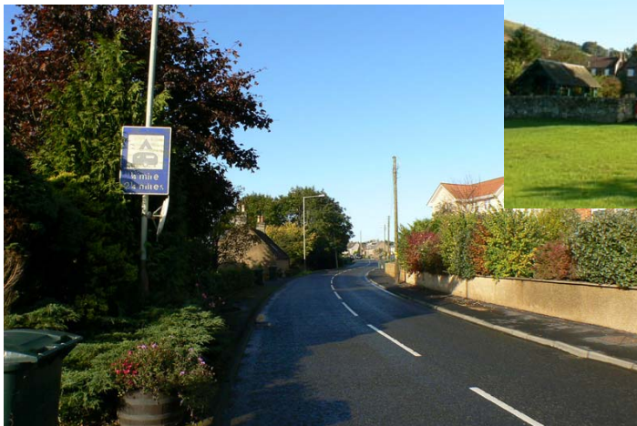
Entrance from the east
