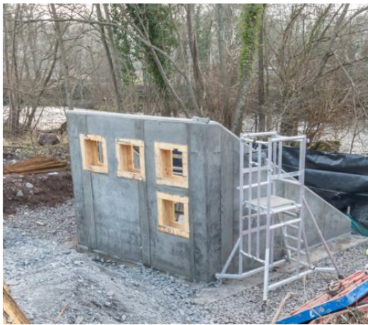
18. Trout Farm – pumping station outfall (the gaps are for pipes).
