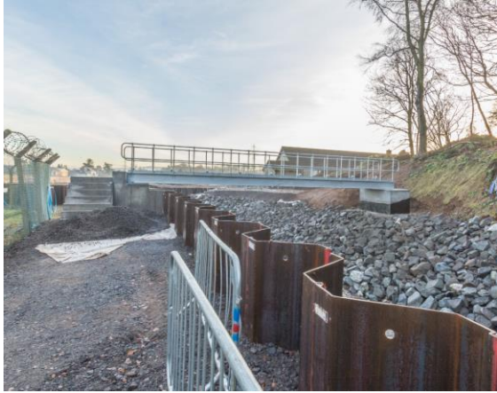
88. Vector – new service bridge under construction.
