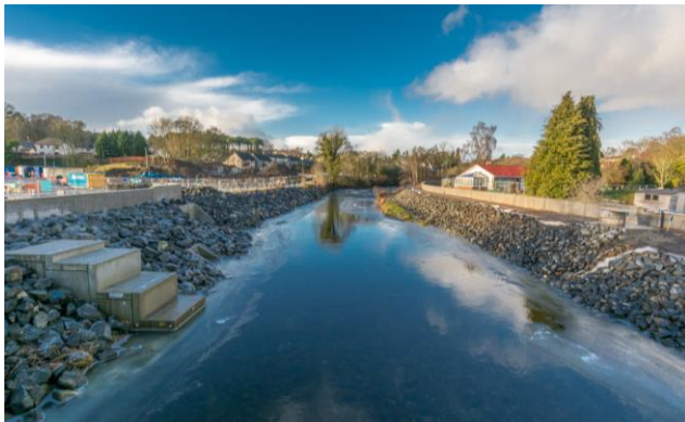
84. Black Bridge – view looking upstream of Black Bridge
