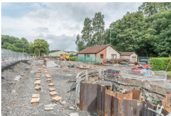
61. Lochty Park – foundation piles completed and ready for abutment.
