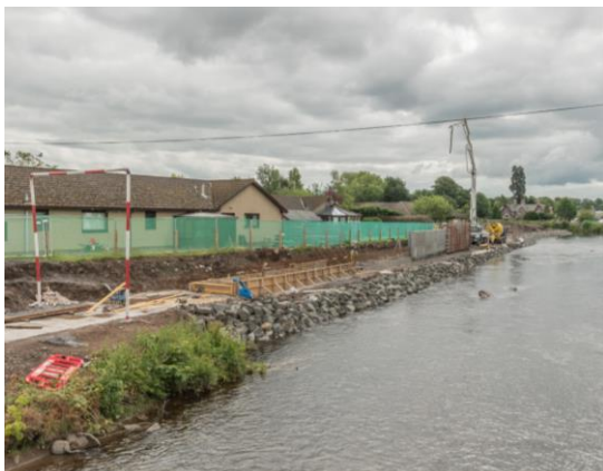
49. Deer Park – construction of flood walls and erosion protection.
