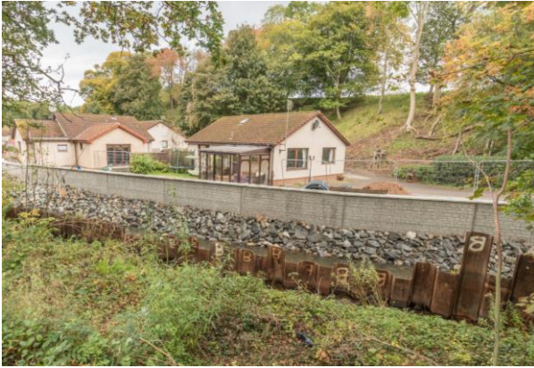
69. Lochty Park – completed flood wall
