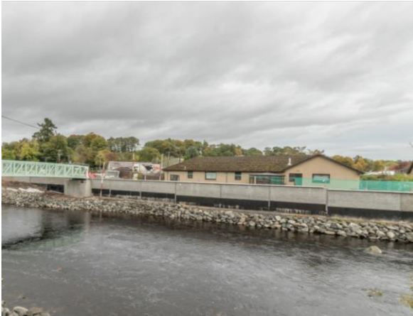
71. Deer Park – completed flood wall
