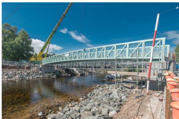
60. Black Bridge – placement of new 'Black Bridge' adjacent to relocated original (see photo 31)
