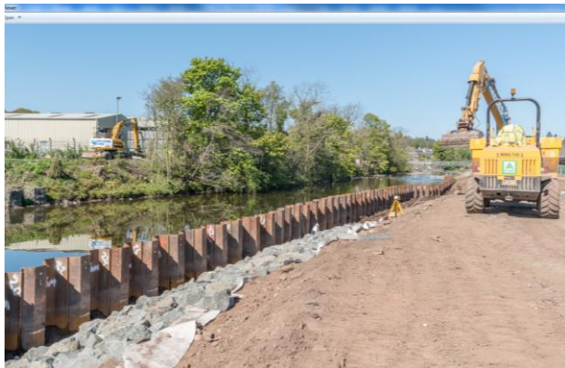
36. Deer Park – installation of erosion protection behind temporary sheet piling.
