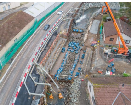
73. Lochty Park – aerial view of Lochty Bridge works.
