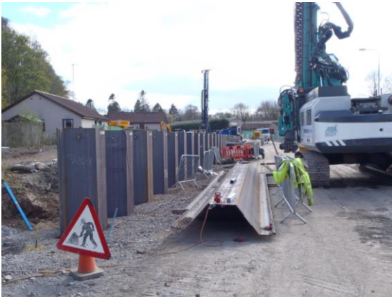
30. Lochty Park – installation of sheet pile flood wall.
