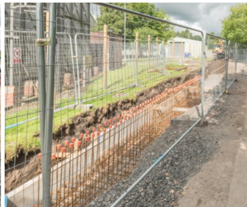
54. Vector/Access road to Low's Works – construction of flood wall
