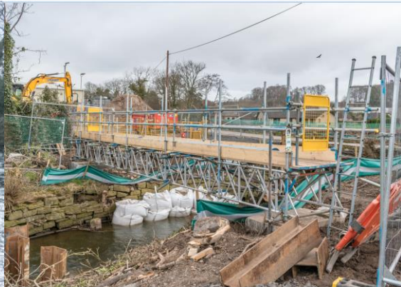
21. Low's Works Cottages/Brockhill – installation of temporary service diversion bridge.
