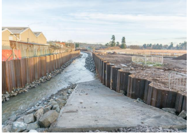
89. Puddledub – one of several access points to the river for maintenance purposes.
