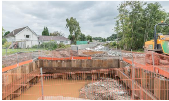
64. Trout Farm – excavation for pumping station.
