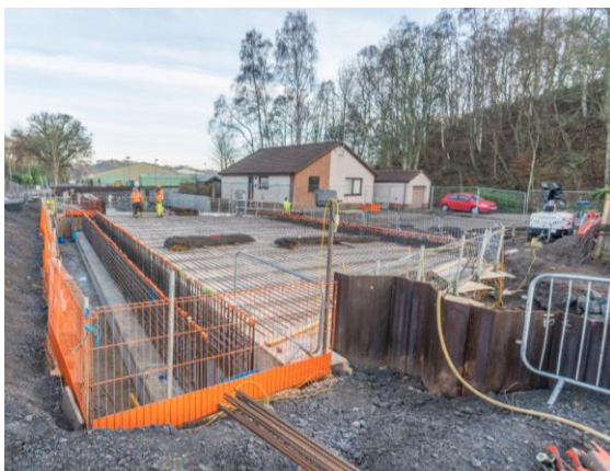
86. Lochty Park – bridge abutment and deck reinforcement being placed.
