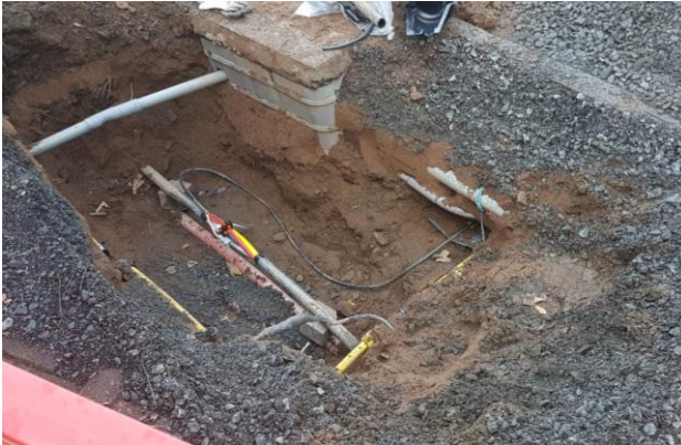
6. Lochty Park – public utility diversion works.
