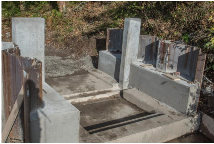
75. Trout Farm – reinforced concrete structure for Tilting Weir.
