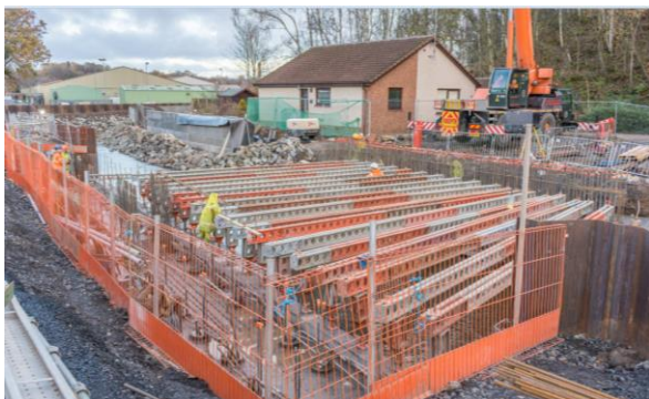
80. Lochty Bridge – supports placed for the new concrete deck.
