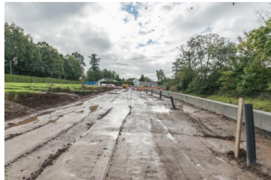
66. Trout Farm – flood wall complete and reinstatement of fish ponds commenced.
