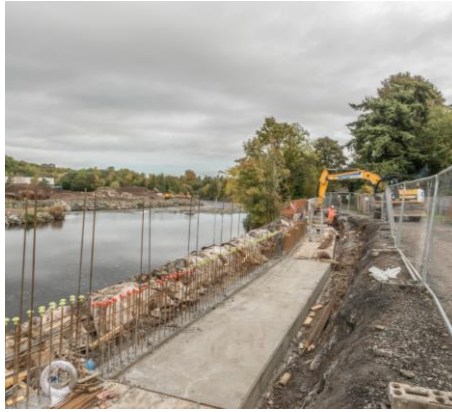
70. Lows Works Cottages – flood wall base complete. Stem reinforcement being erected.
