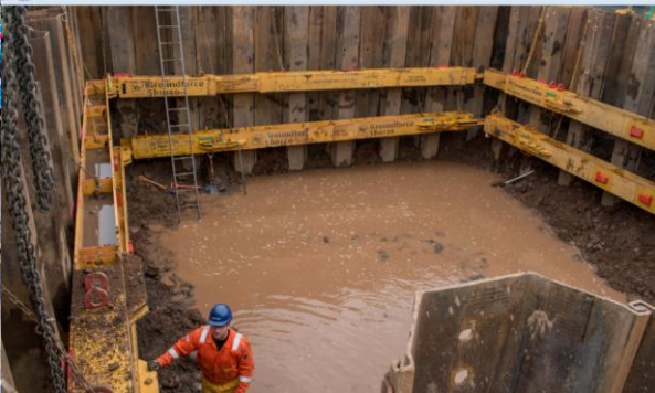
15. Vector – installation of temporary sheet piles to construct pumping station chamber.
