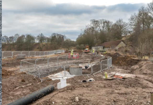
7. Puddledub/Brockhill - construction of drainage system for new access road.
