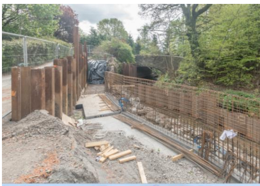
39. Heron Lodge – construction of flood wall stem reinforcement.
