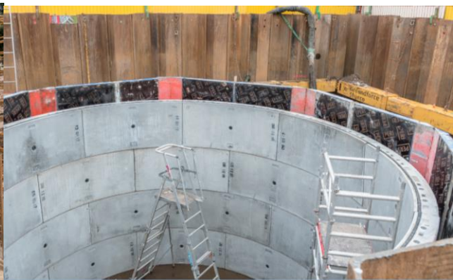
25. Vector – construction of pumping station chamber with concrete segments.
