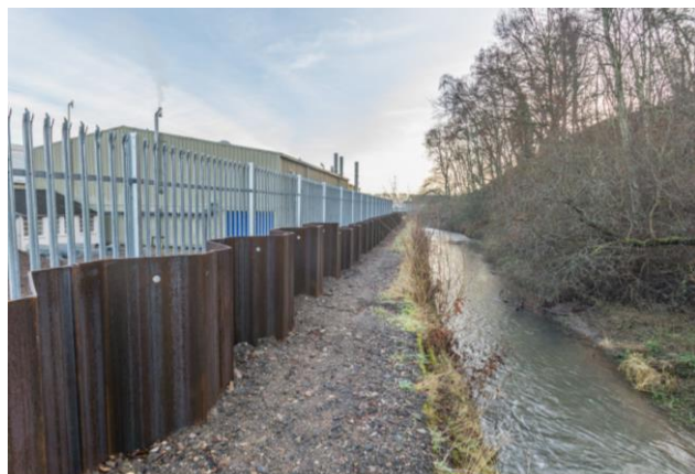
87. Vector – Vector security fencing and Sheet pile flood defence wall complete.
