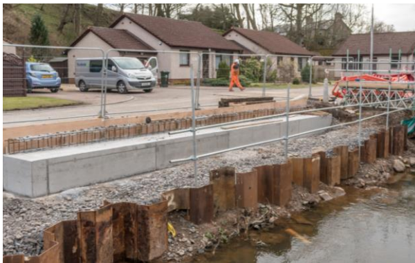
22. Lochty Park – construction of the temporary bridge reinforced concrete foundation.
