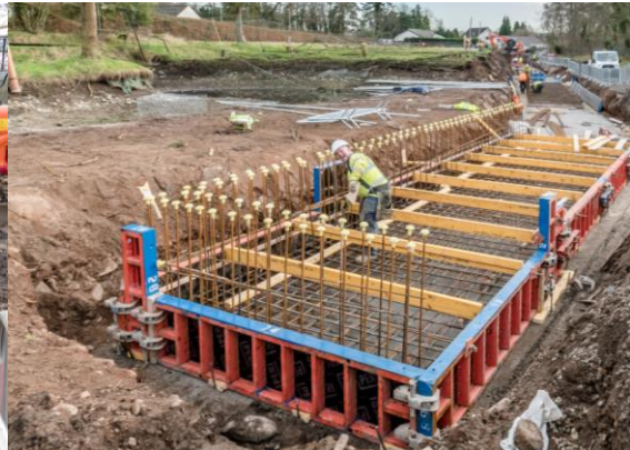
9. Trout Farm – erection of reinforcement and shuttering for flood wall bases.
