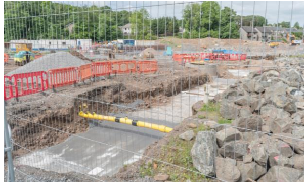
44. Cricket Pitch – commencing flood wall construction.
