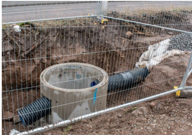
13. Cricket Pitch – construction of drainage system.
