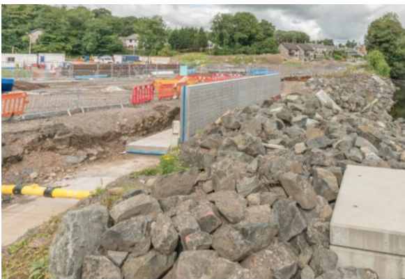
55. Cricket Pitch – construction of flood wall.
