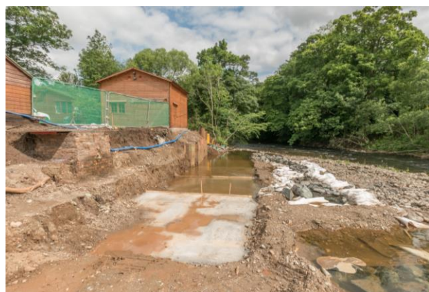
50. Cragneuk – commencing construction of flood walls.
