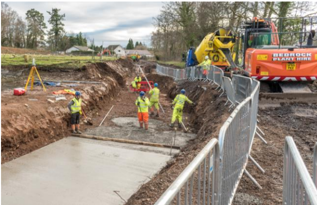
8. Trout Farm – commence construction of flood wall base.
