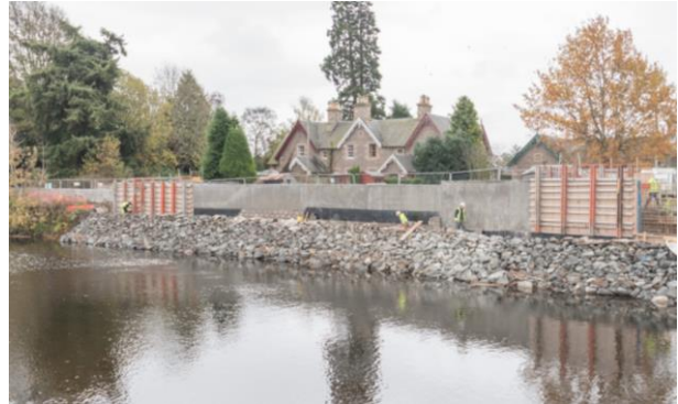
77. Lows Works Cottages – flood wall stem complete
