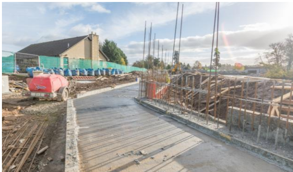
78. Deer Park – flood wall base complete and stem reinforcement being erected.
