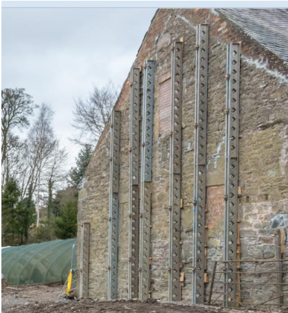
12. Trout Farm – temporary bracing of building during the works.
