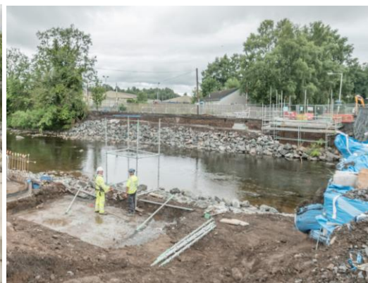
56. Black Bridge – commencing new bridge foundations.
