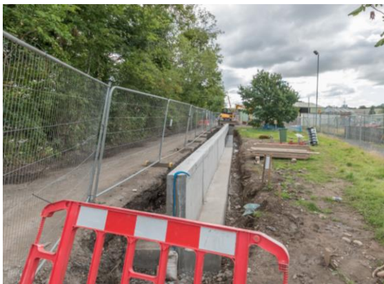
59. Vector – continuation of flood walls along private access road to Lows Works Cottages etc.
