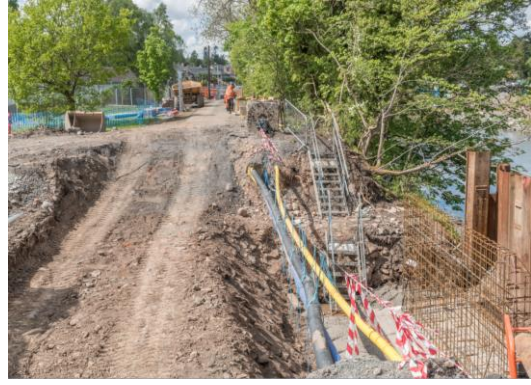
42. Vector – construction of pumping station outfall opposite Deer Park.
