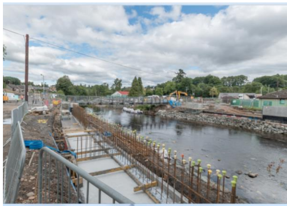
58. Deer Park – construction of flood walls and erosion protection.
