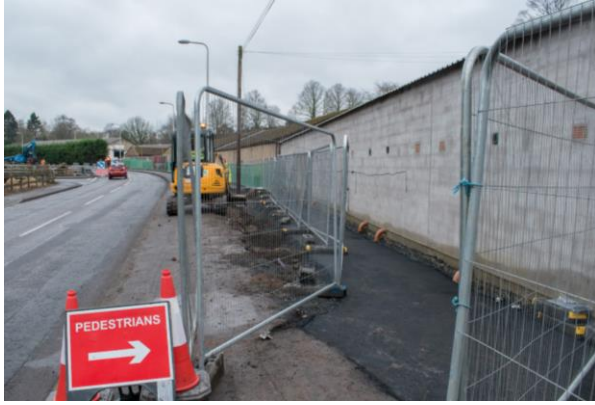
16. Lochty – construction of temporary pedestrian access.
