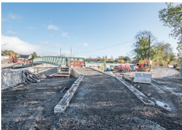
74. Black Bridge – access ramps being built.
