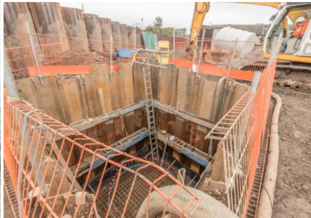
72. Brockhill – base reinforcement being erected for pumping station.
