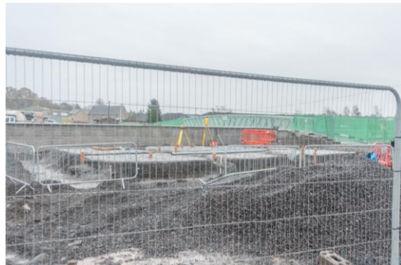
81. Cricket Pitch – foundation of new Community Pavilion being constructed.
