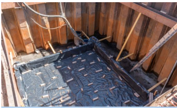
37. Craigneuk – inside excavation for construction of pumping station reinforced concrete base.
