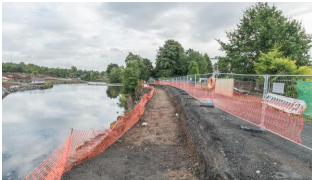
65. Lows Works Cottages – excavation complete for flood wall.
