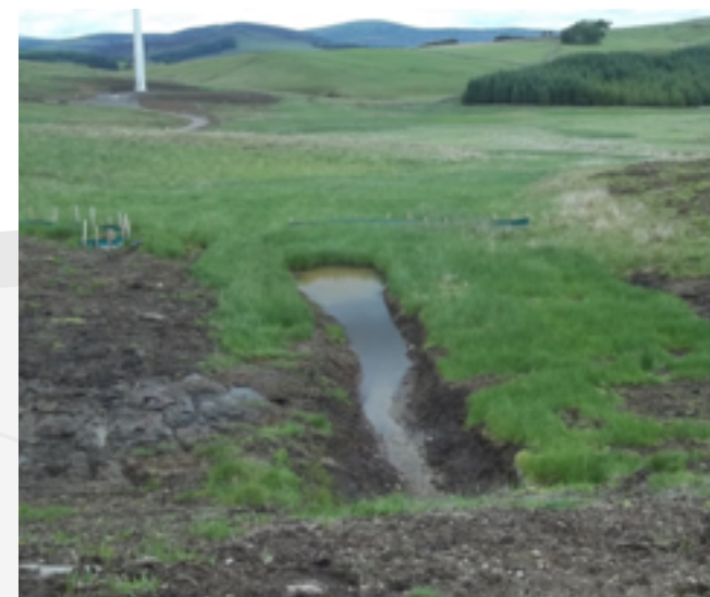
Managed dispersal of silted water through adjacent grasslands.
