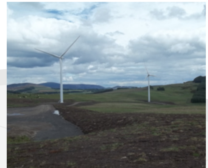
Reinstatement and ground profiling using turfs around tracks and crane hardstandings
