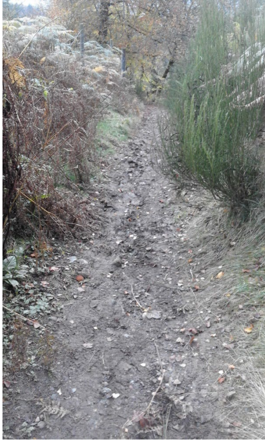
Erosion on path on steep gradient (along eastern boundary). Caused by combination of foot traffic, horses and surface water run off
