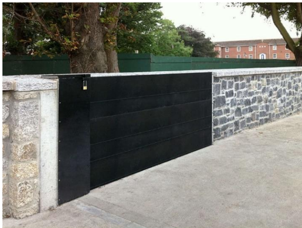
Image 9.3 Example vehicle access flood gate
