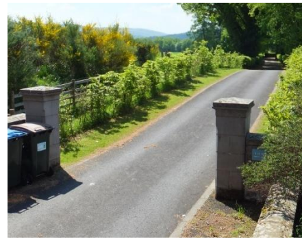
Vehicle access ramp
