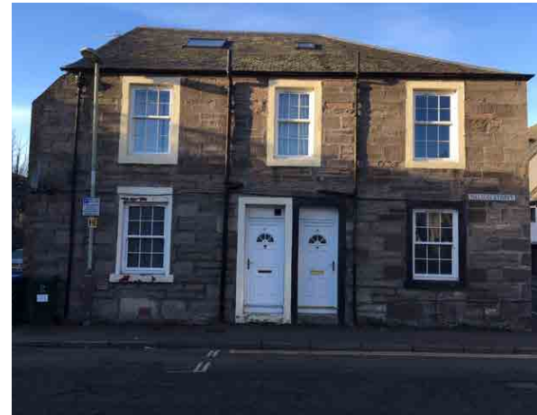
The choice of colours on door and window frames impacts on the original symmetry of the building
