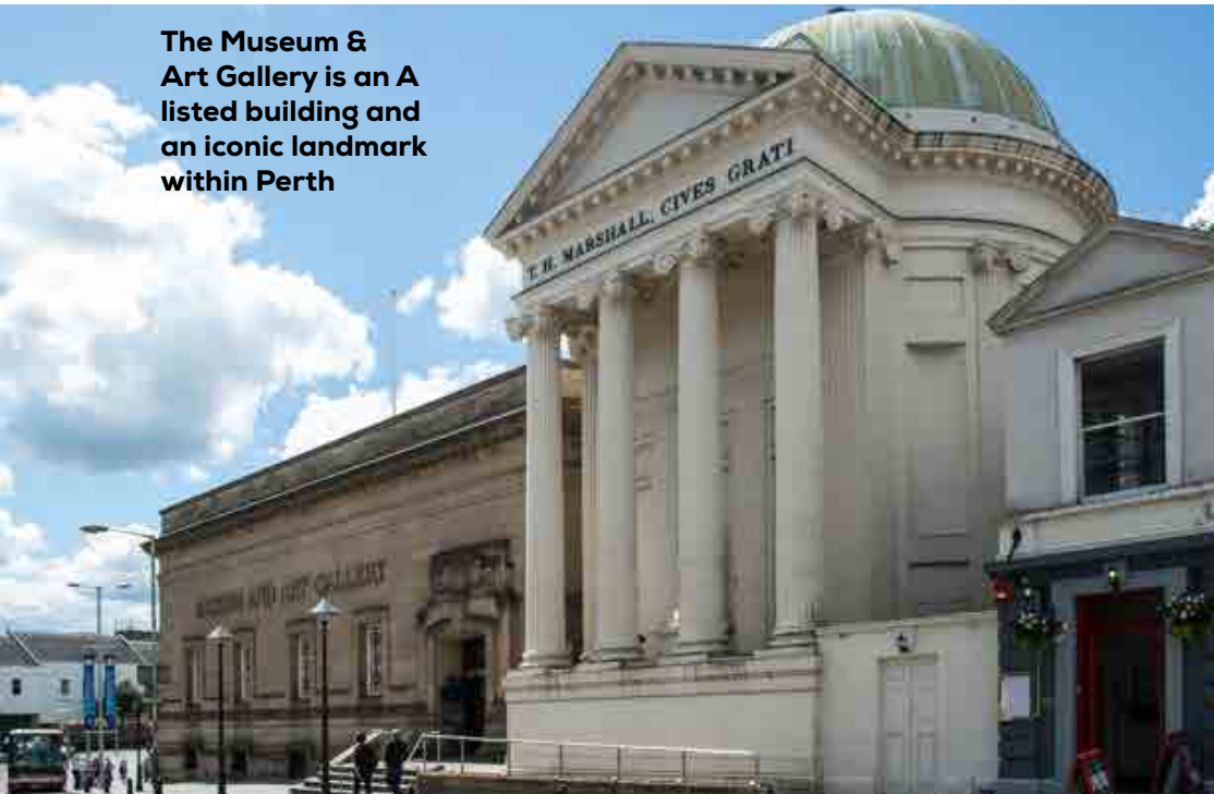
Perth Concert Hall has created a new focal point within the city
