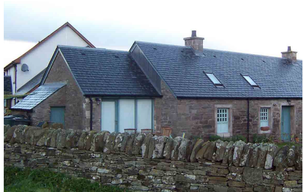
Modern extension on traditional building reflecting the simple vernacular of the original building
