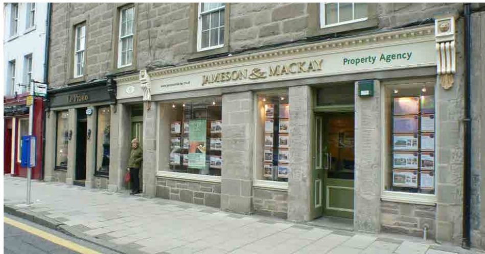
New lettering sensitively designed and installed on historic fascia, both in scale and in keeping with shopfront
