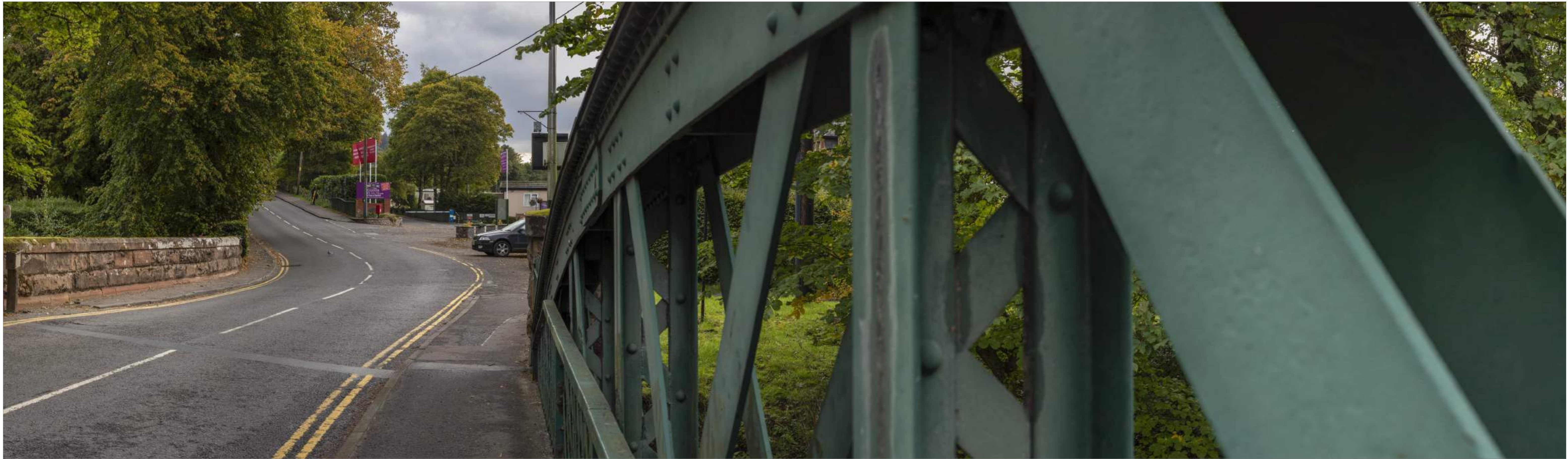
Comrie Flood Protection Scheme - Viewpoint Figure 5.6.7.2- Viewpoint 7: Lednock Bridge
