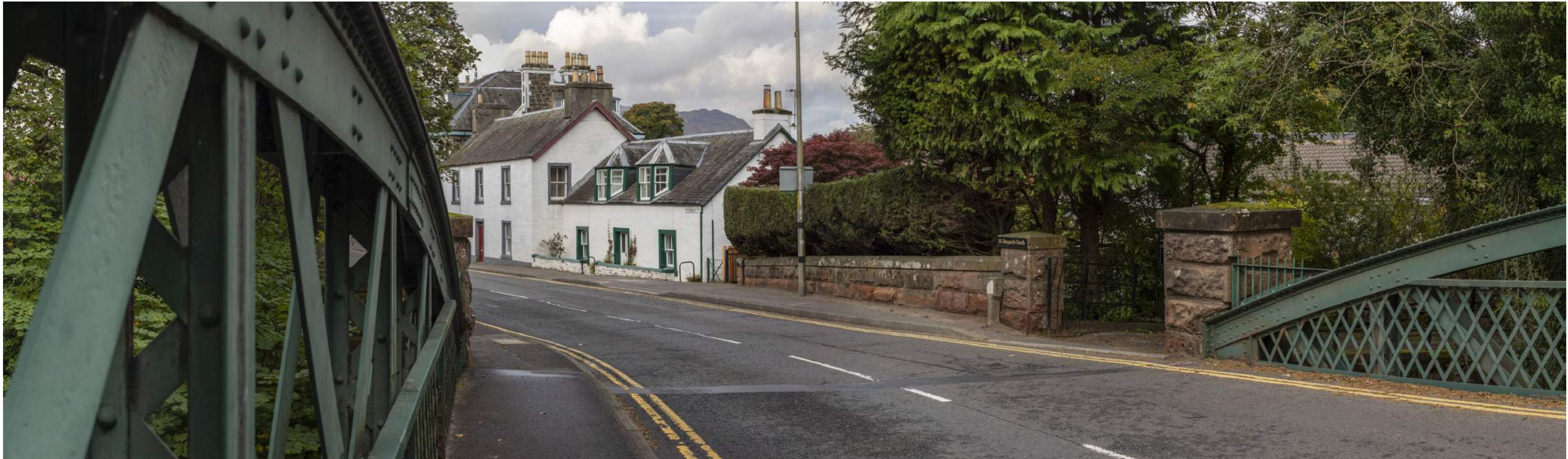
Comrie Flood Protection Scheme - Viewpoint Figure 5.6.7.4- Viewpoint 7: Lednock Bridge
