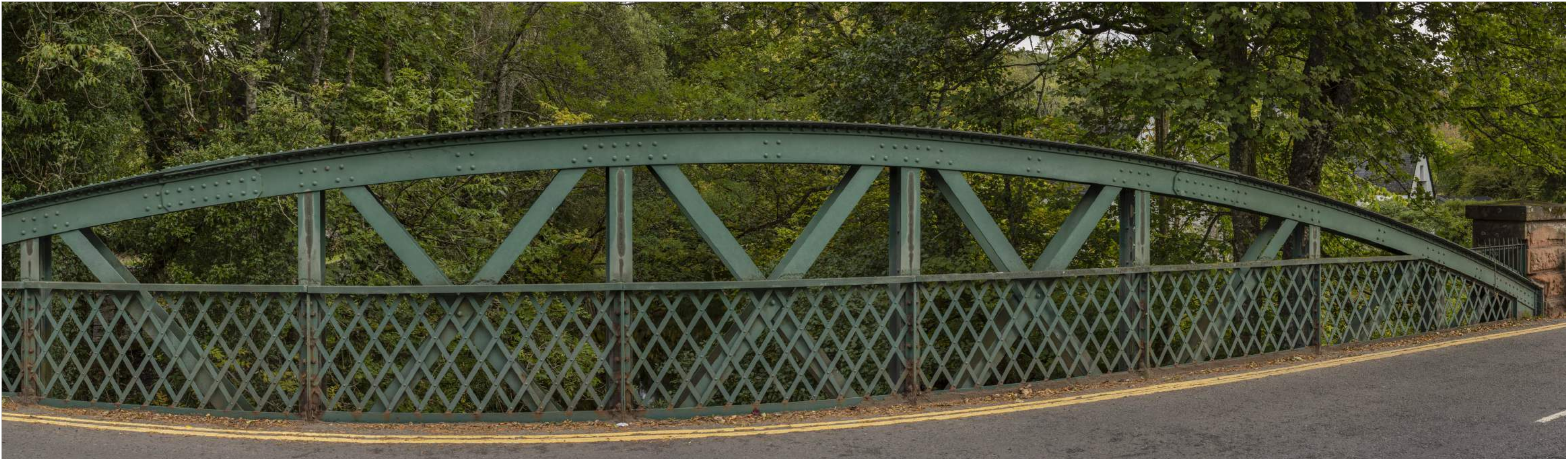
Comrie Flood Protection Scheme - Viewpoint Figure 5.6.7.3- Viewpoint 7: Lednock Bridge
