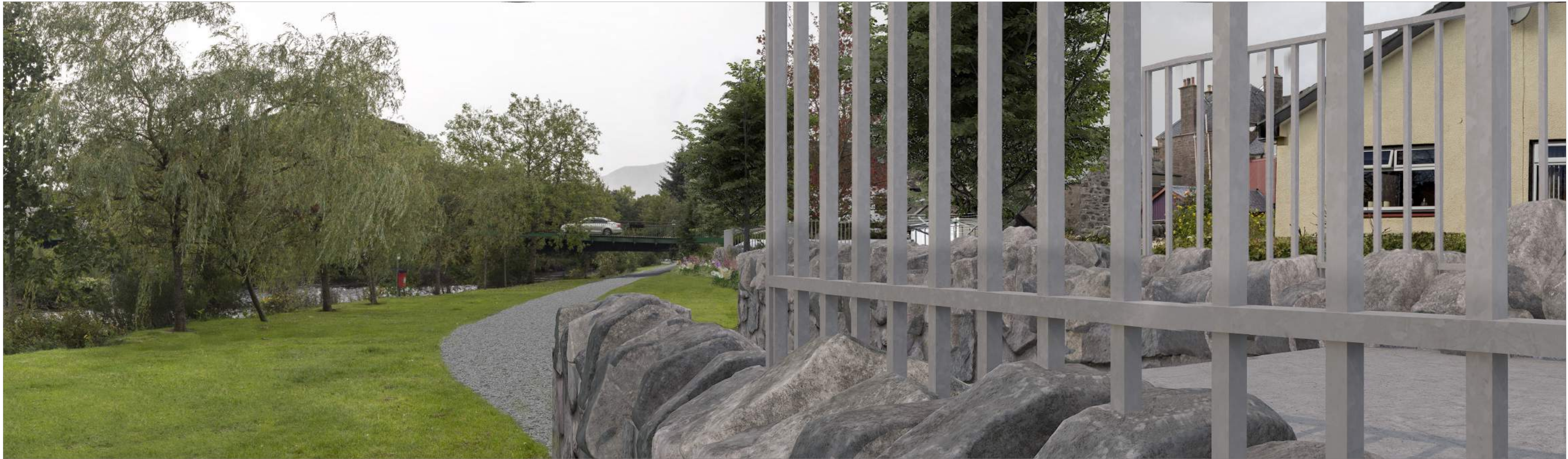
Comrie Flood Protection Scheme - Photomontages Figure 5.6.5.3.3 - Viewpoint 5: Open Space North of the River Earn
