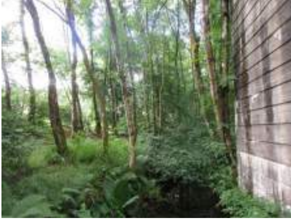
Rail Embankment South view west along mill lade adjacent tree 1231
