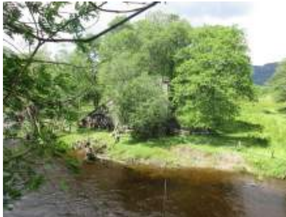
Mid Tullybanochter Embankment North view from opposite bank
