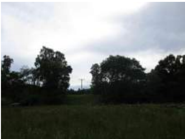
Mid Tullybanochter Rail Embankment north with gap for former bridge viewed from field to east
