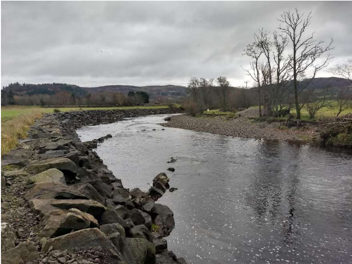
Figure 3-5: Photo showing bank protection and J-vanes at Ruchilside
