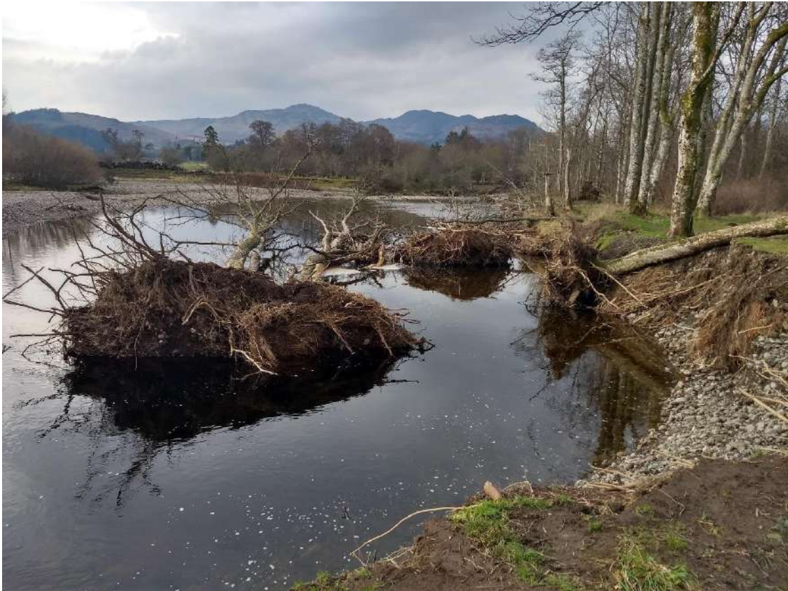
Figure 3-14: Photo of severe bank erosion downstream of the failing rip-rap bank protection at the outer meander bend at the Field of Refuge.
