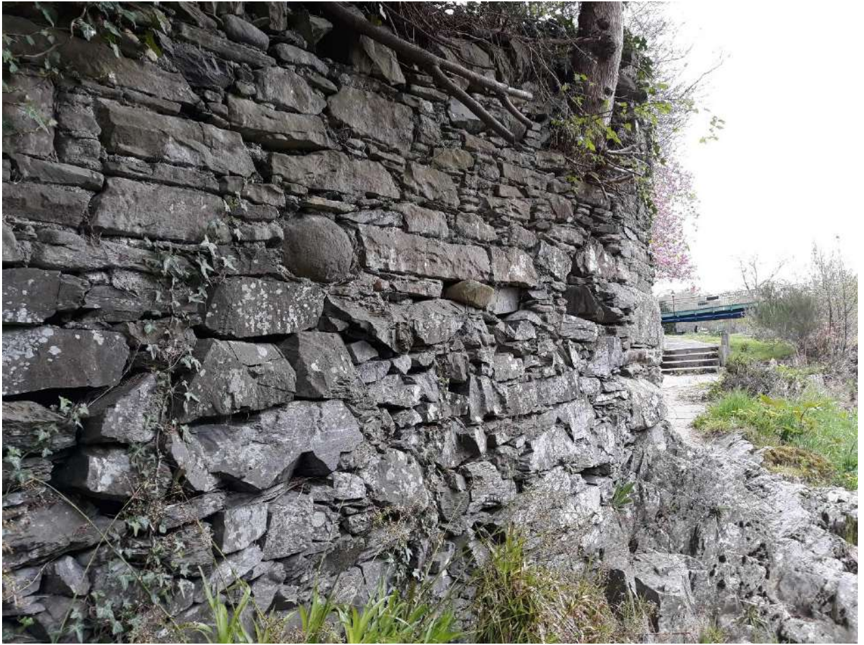
Figure 4. S3 – Dry stone wall with gaps between brickwork presenting bat roosting opportunities.
