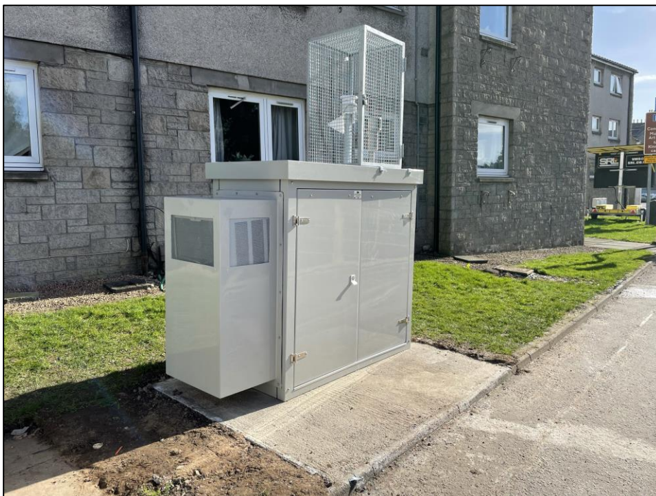
Relocated RTM in place at Bridgend Perth
