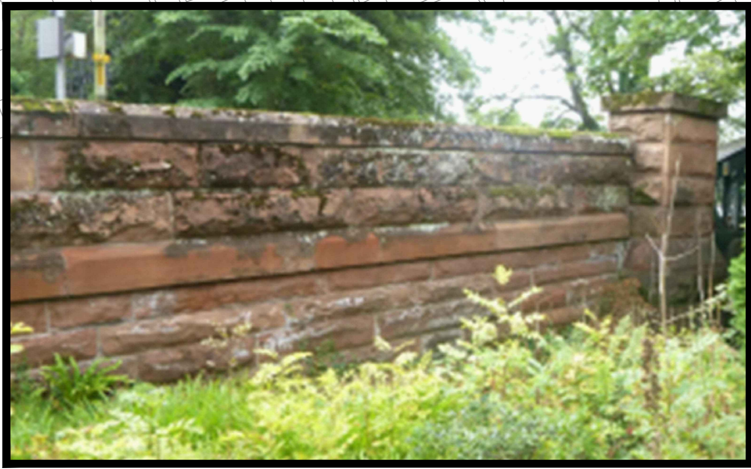
FINISH TYPE F2: RED ASHLAR SANDSTONE CLADDING
