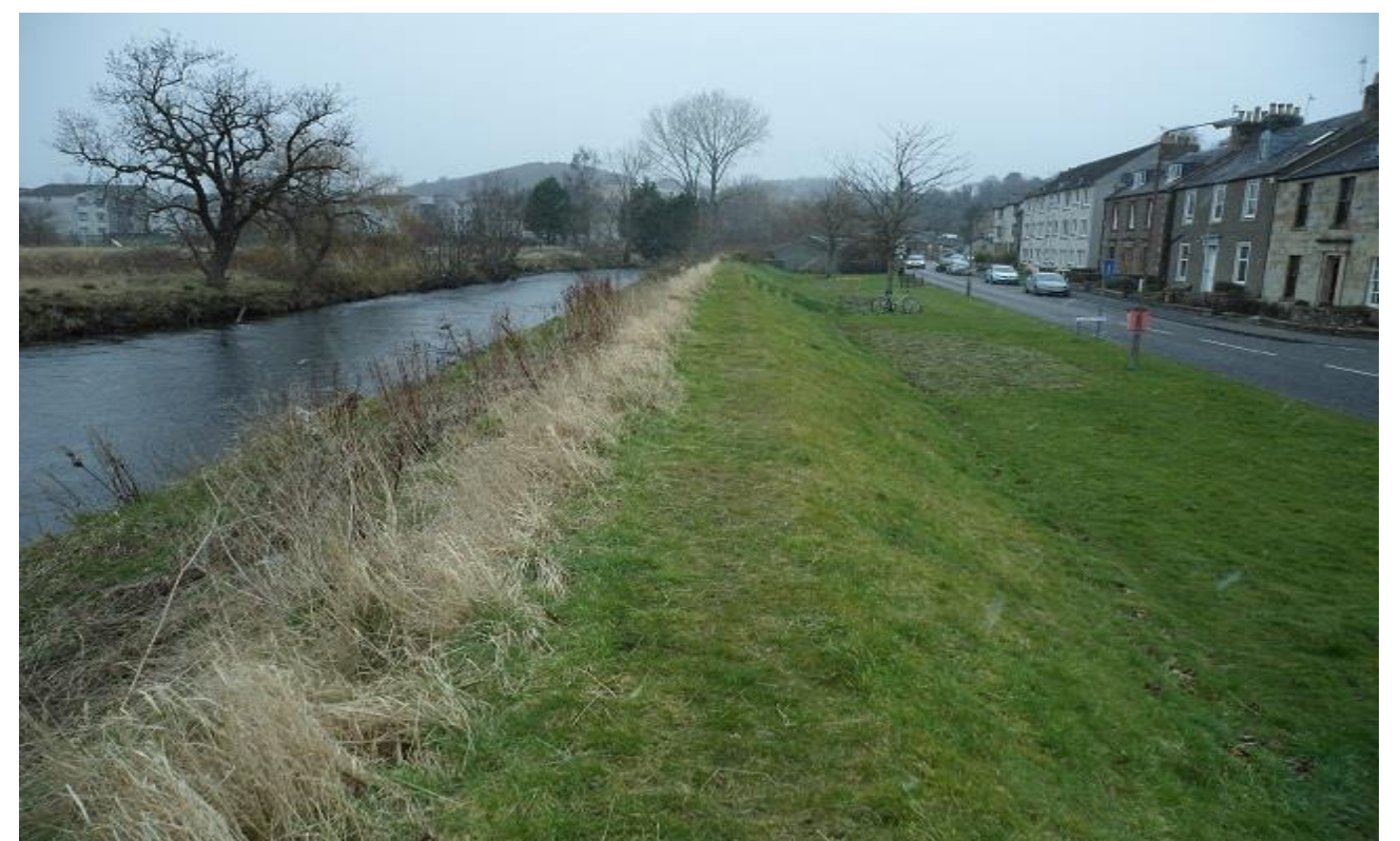
Typical flood embankment
