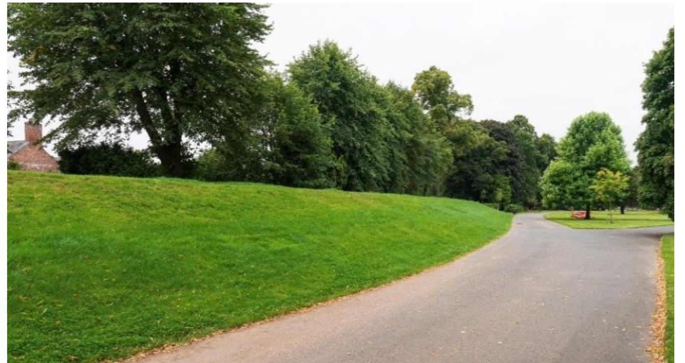
Typical flood embankment
