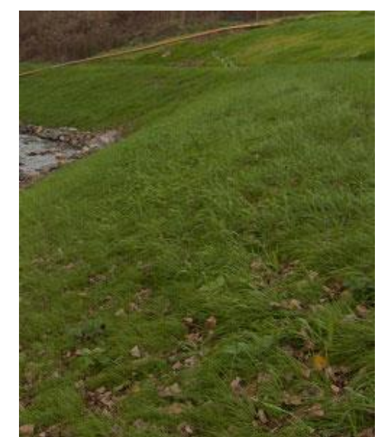
Example of flood embankment with coir matting erosion protection during construction and post grass establishment
