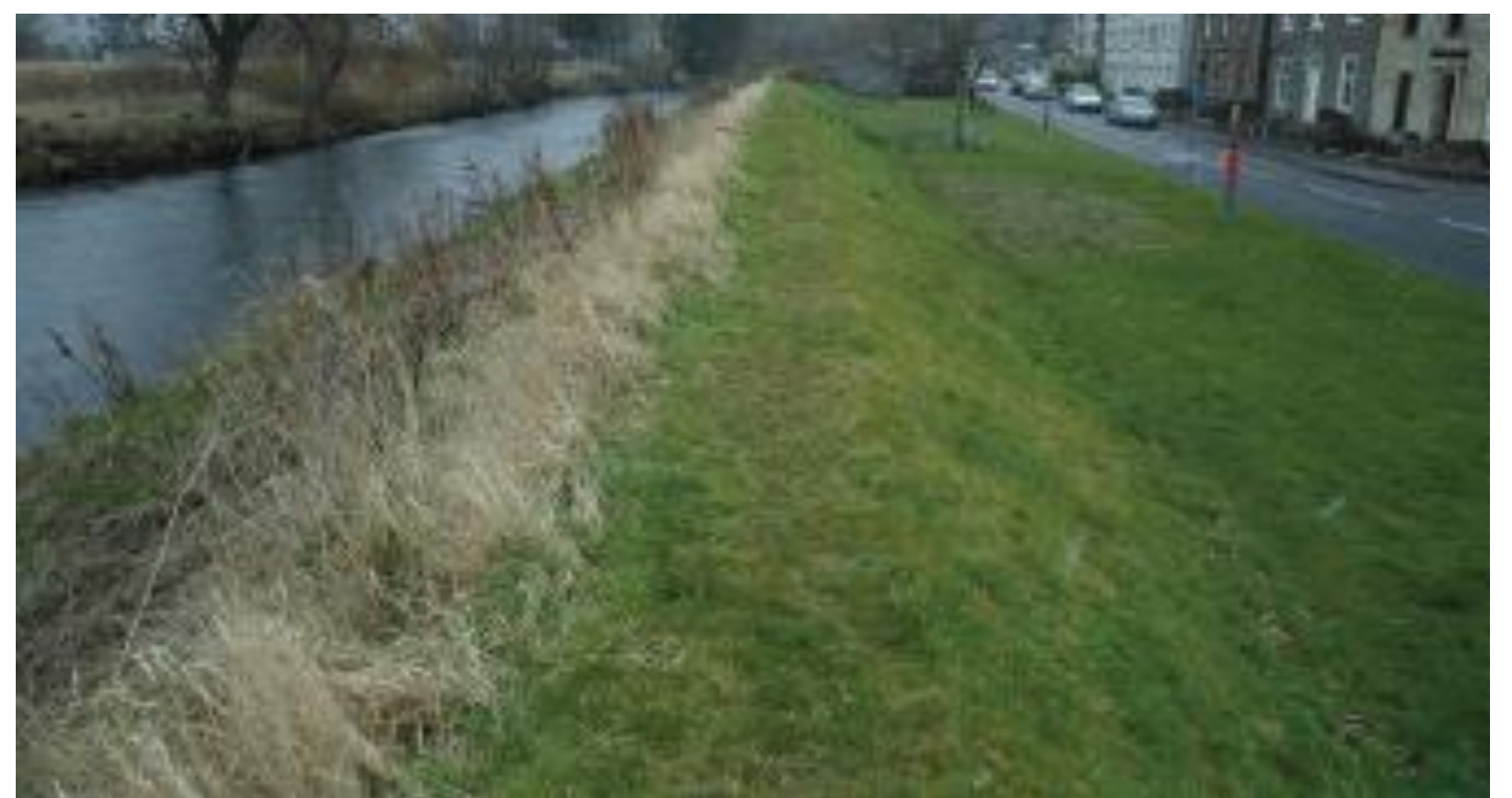
Figure 10 Example of a Flood Embankment
