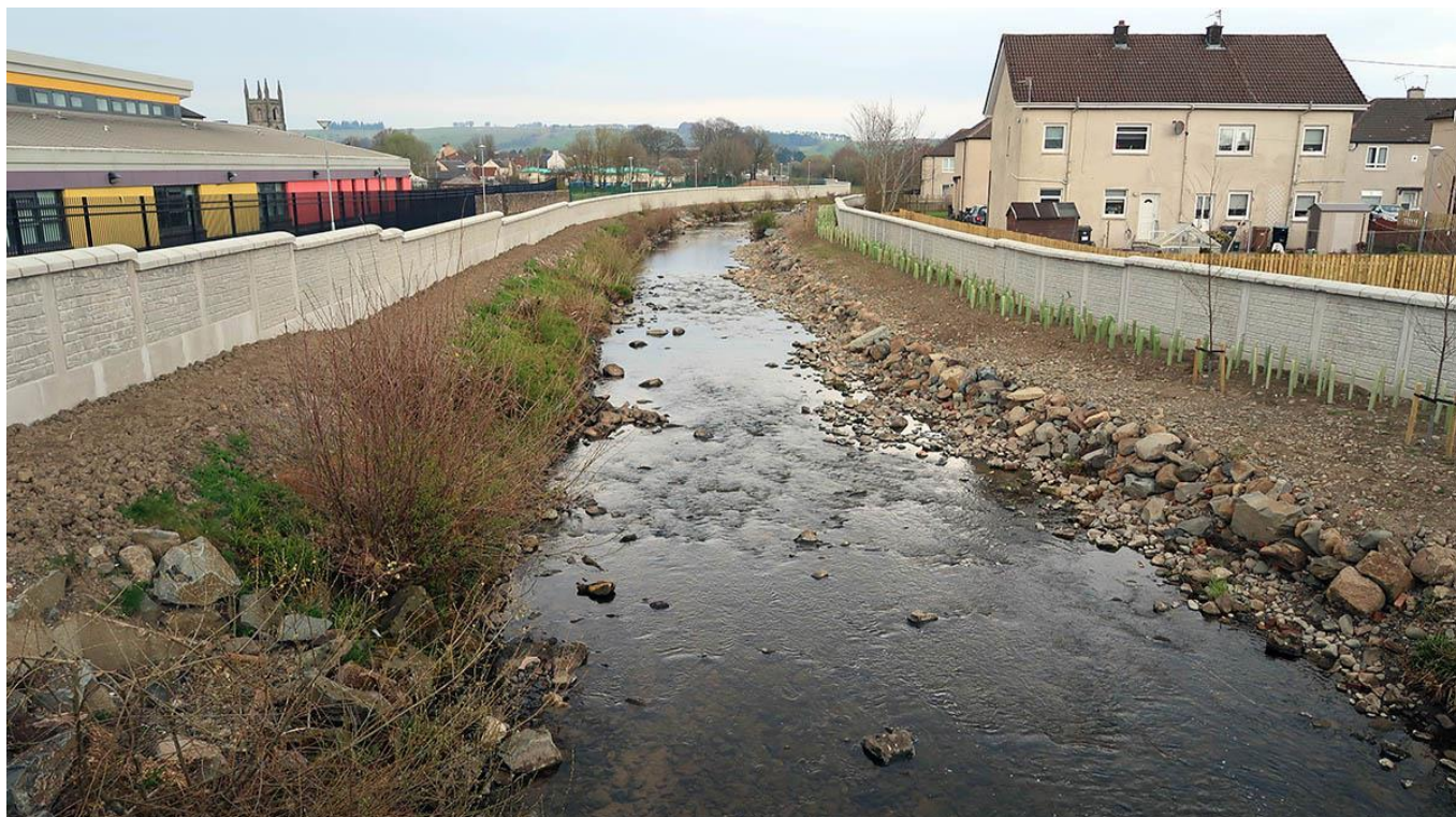
Figure 9 Example of a Flood Wall
