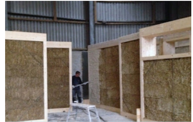
Modcell Panel System Timber framed panel infilled with compressed straw bales
