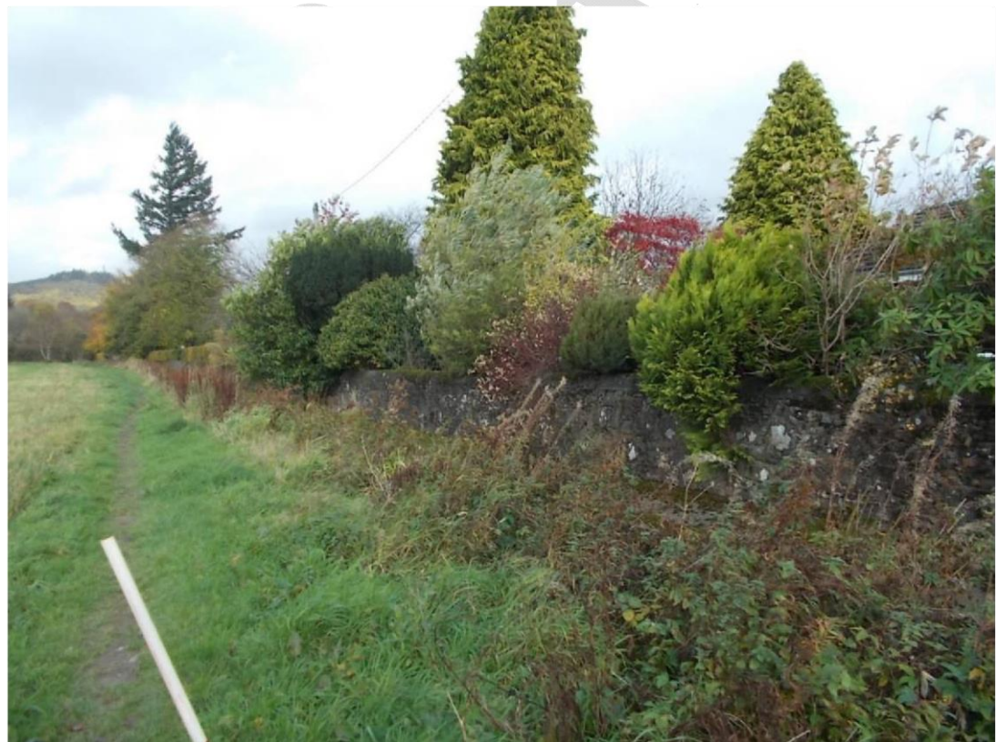
Photograph 8 – Concrete base with concrete/masonry stem
