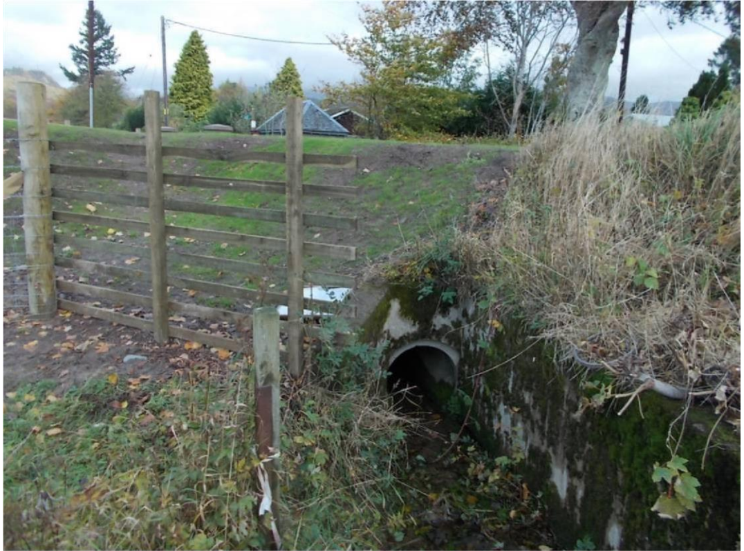
Photograph 5 – South end of the pipe
