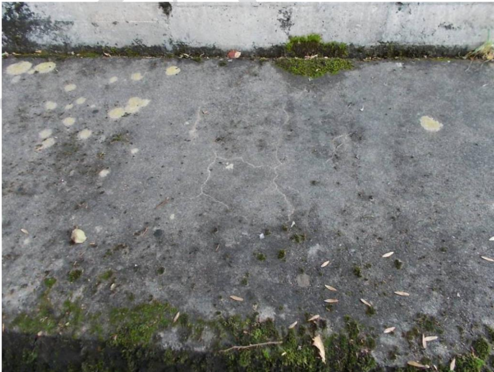
Photograph 25 calcite deposits and multiple cracks on base of concrete.
