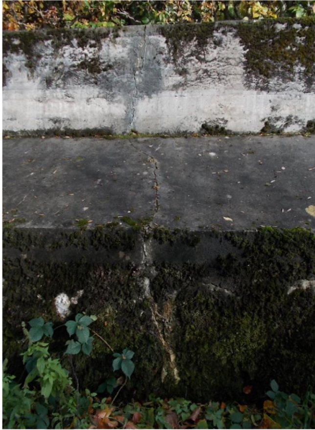
Photograph 25 calcite deposits and multiple cracks on base of concrete.
