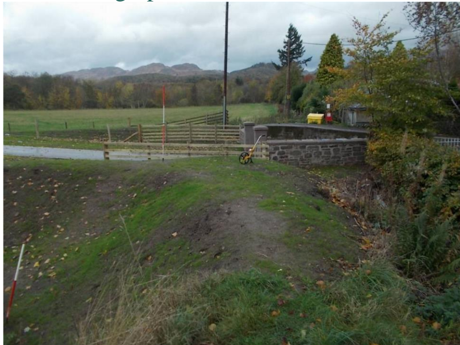
Photograph 1 – Earth bund looking north
