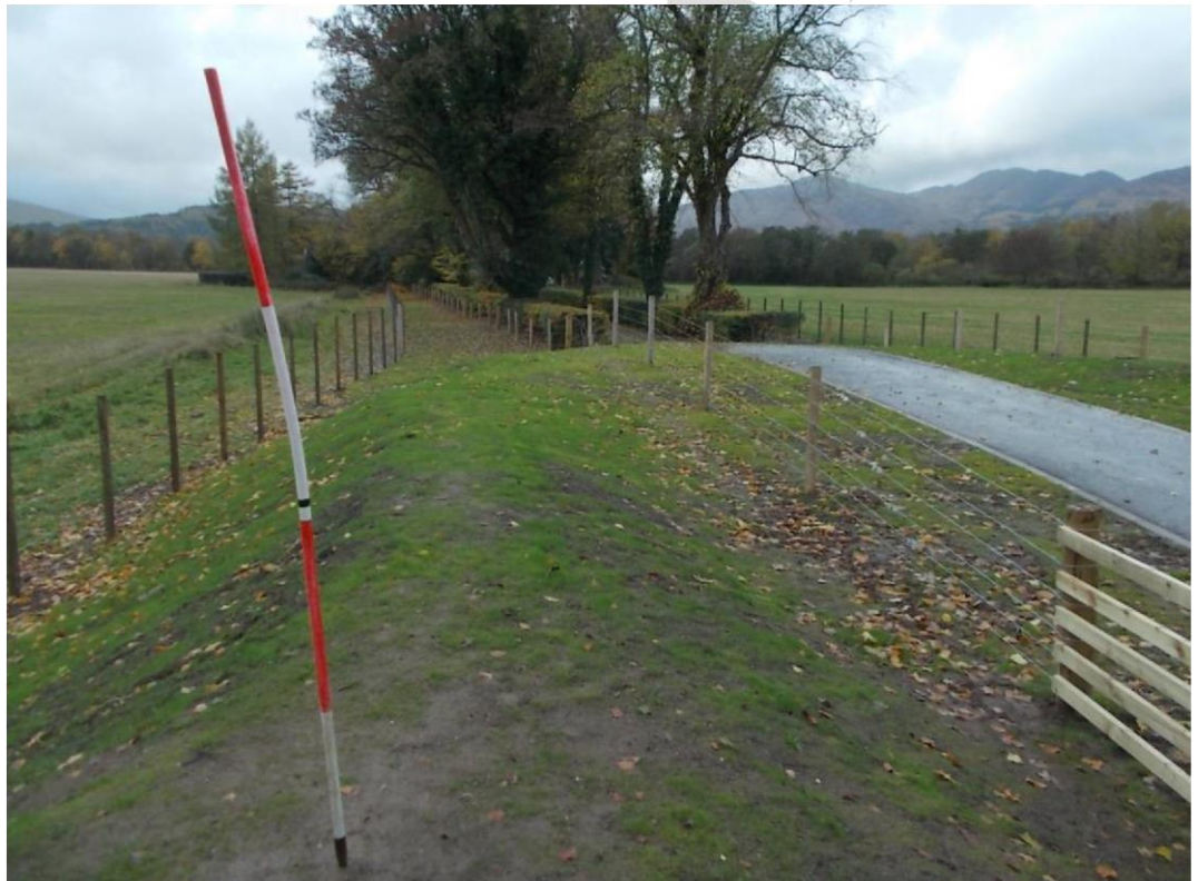
Photograph 6 – looking west towards Tomnagaske House
