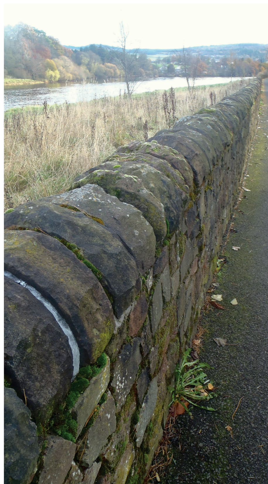
Figure 5: Typical Flood Protection Wall (North Muirton, Perth).
