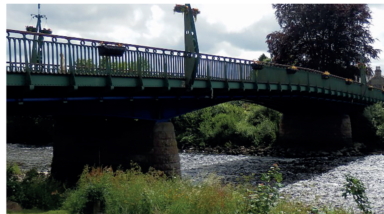
Figure 23: Dalginross Bridge over the River Earn.
