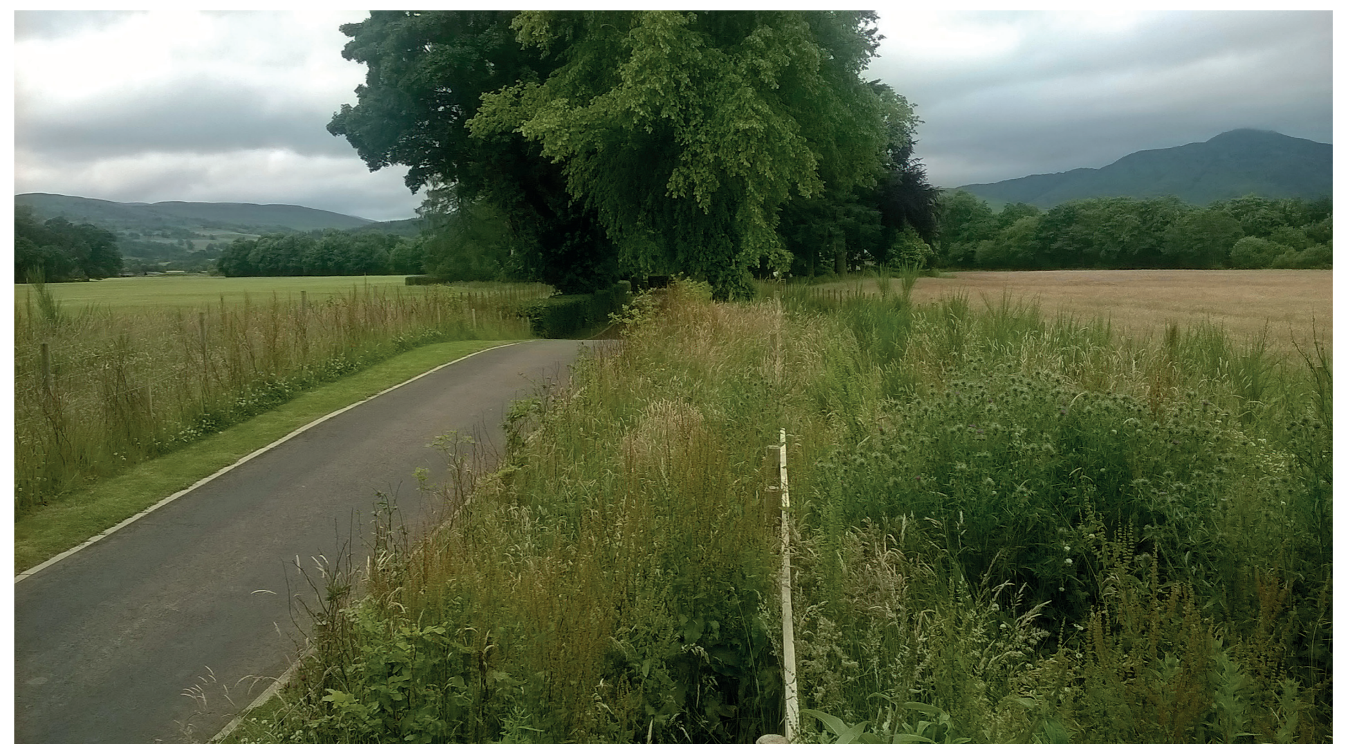
Figure 3: Flood protection works on the Water of Ruchill (2013).
