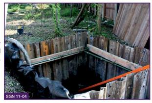
Alternatives to thrust boring are to hand-dig broken or continuous trenches, so that roots can be retained (with the service ducting threaded beneath). Note the ground protection boards with soil piled on top on the left.
