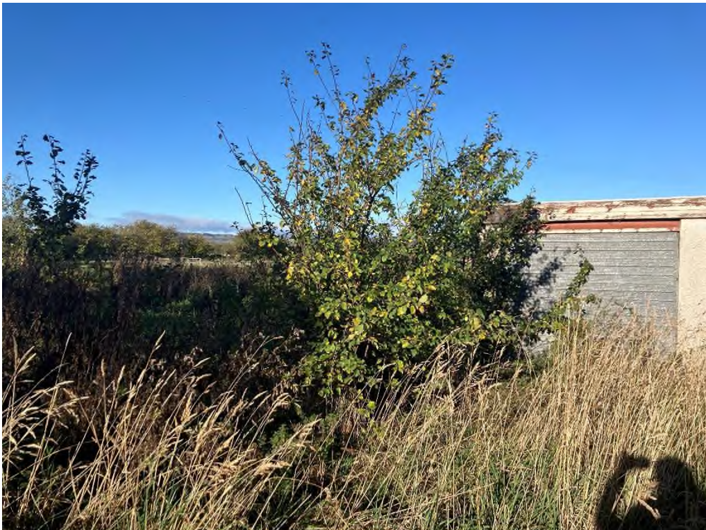
Figure 2: Overgrown Vegetation around Derelict Building
